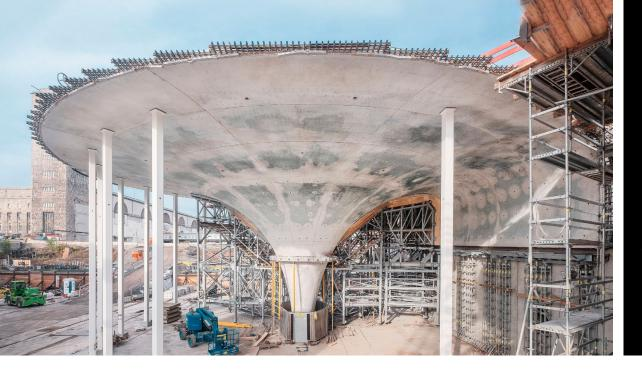
Concreted cup support for the platform hall of the new Stuttgart underground station. © Ed. Züblin AG / Achim Birnbaum
