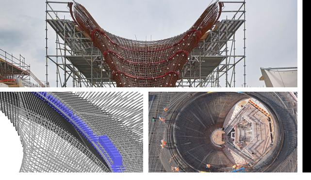
Picture above: and right: Reinforcement of a chalice-shaped column of the new Stuttgart underground station © Ed. Züblin AG / Achim Birnbaum
